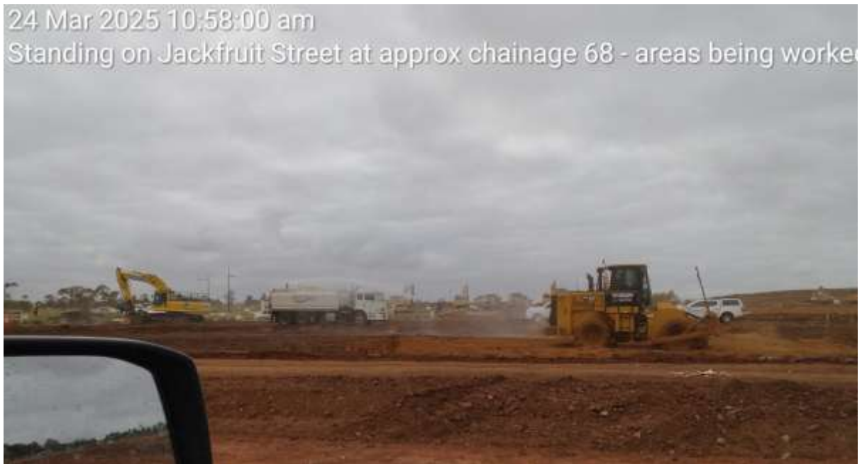
Figure 2: Fill Being Moisture Conditioned During Compaction Process (Source: C&T)
