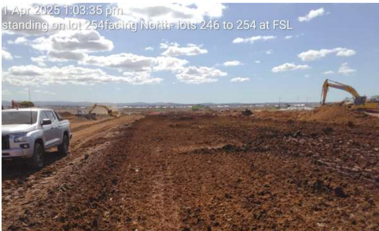
Figure 3: Completed Fill Placement on Lots 246 - 254 (Source: C&T)
