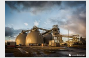
BIOMASS STORE & FUEL HANDLING
