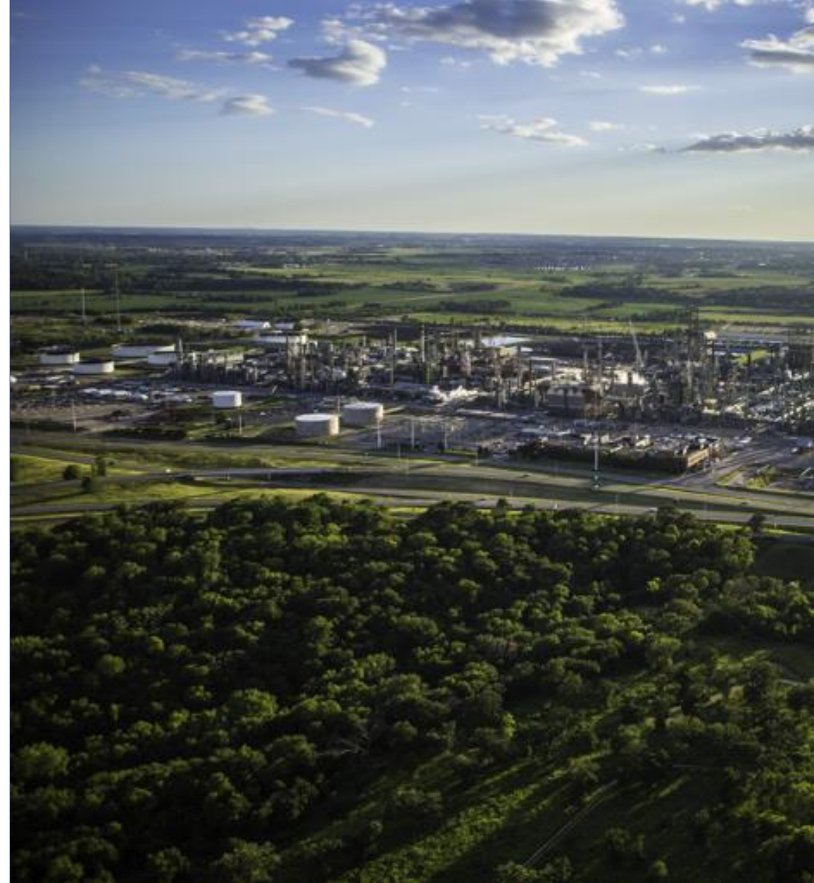
Pine Bend Refinery Rosemount, MN
