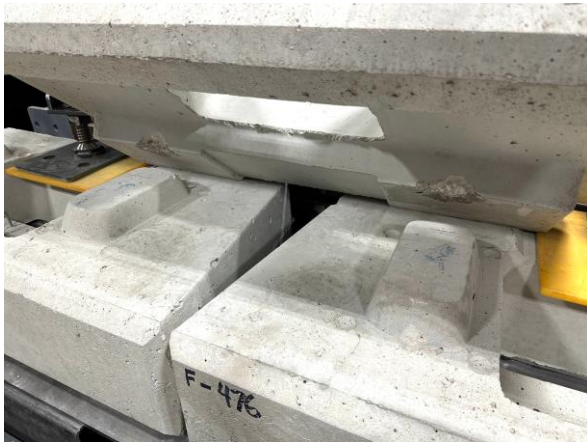
Figure 3 – Groove crushing at shear knobs
