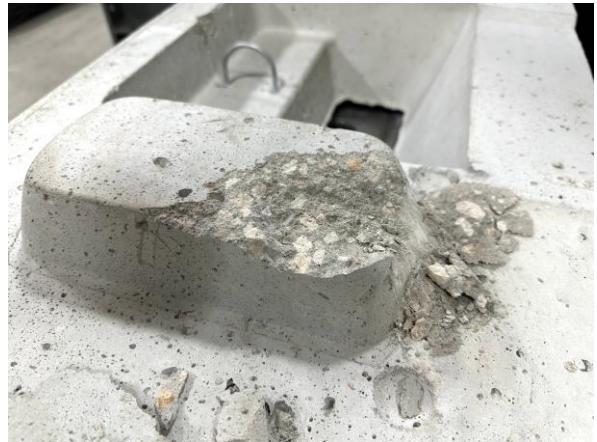
Figure 4 – Broken shear knob
