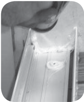
Caulking of base channel
