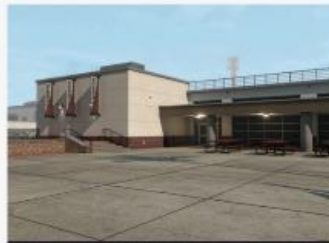
CAMPUS - ENTRY 3 Facing Cafeteria
