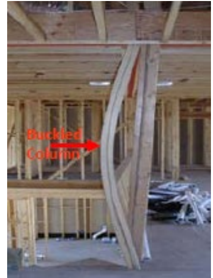
Figure 1: Column Buckling
