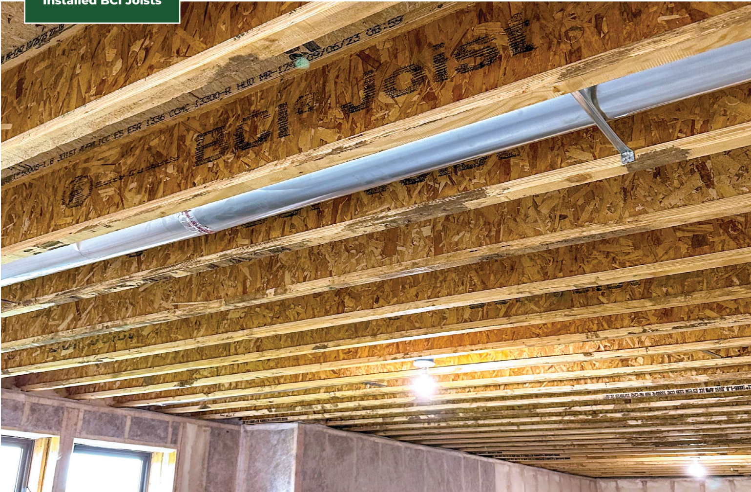
Installed BCI Joists
