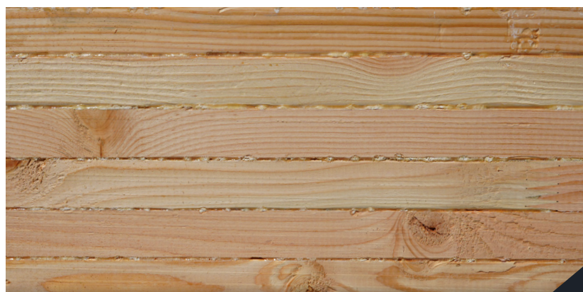
Framing Appearance Beam
