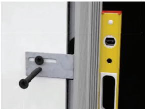
Adjusting and fixing the Frame
