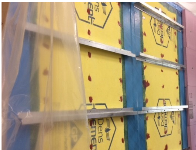
Picture 1: The DensElement ® Barrier System with Z Girts installed with flanges up and down. The Z Girts are installed both tight and spaced from the WRB. Far right test wall shows XPS attached.
