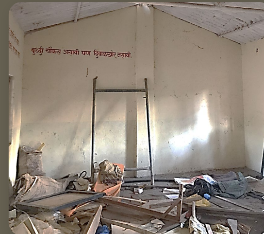
reconstruction of dilapidated classrooms
