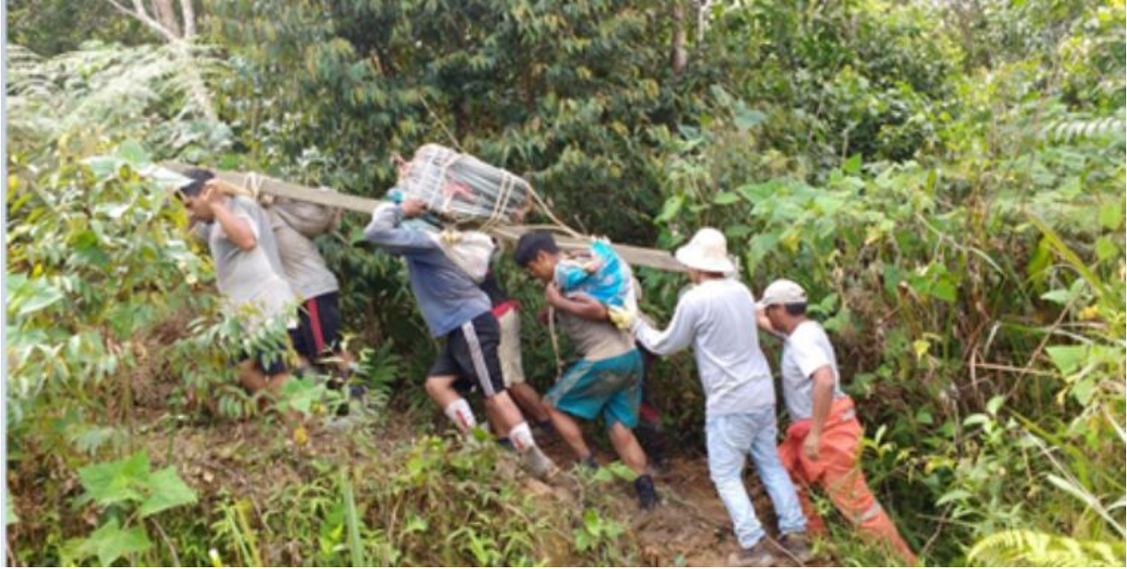
Figure 8 - Picture of construction personnel hand-carrying elements of the radio tower and hardware at the Satipo 1 site
